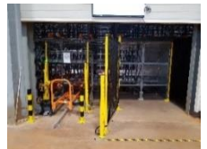
Trolley picking station
